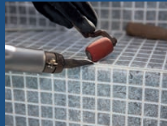
Specialist on-site lining using Ceramics liner material.
